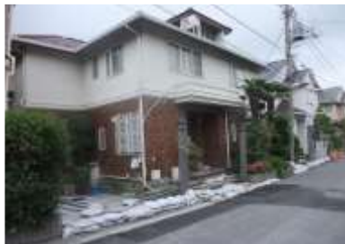
Fig. 14 Settled and tilted houses in Urayasu City
