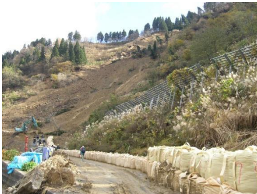
Fig. 7 One of the landslides in former Yamakoshi Village triggered by the 2004 Niigata-Chuetsu earthquake
