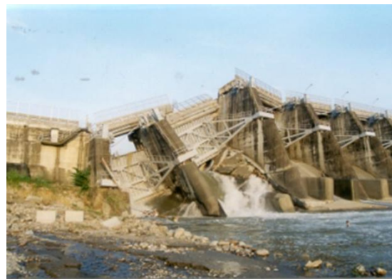
Fig. 21 Sigang Dam that was destroyed by fault uplift during the 1999 Chi Chi earthquake
