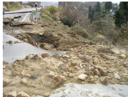
Fig. 8 Coseismic failure of road embankment in the same area as in Figure 7
