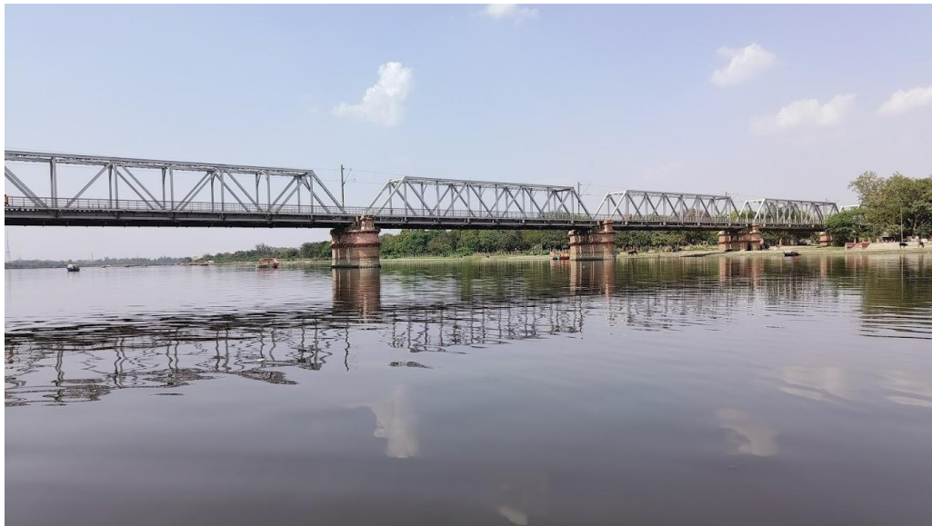
Fig. I1 Railway Bridge over River Yamuna at Mathura
