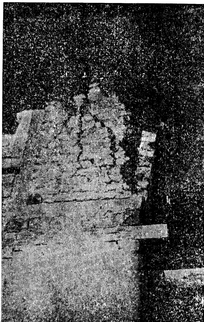
Fig. 8—Buckling of “brick shuttering” at first floor of a brick masonry house at Kolabug.
