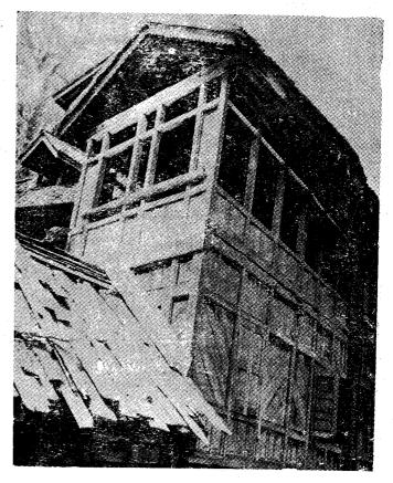
Fig. 48. Building in Mattan having Timber Panelled walls.
