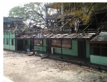
Fig. 5 Assam type house with timber roof trusses
