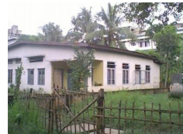
Fig. 8 Confined masonry building with gable end not braced against out-of-plane failure
