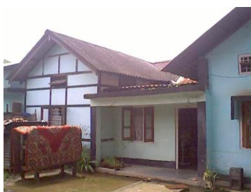
Fig. 4 Assam type house (left) partly replaced with masonry house (right)
