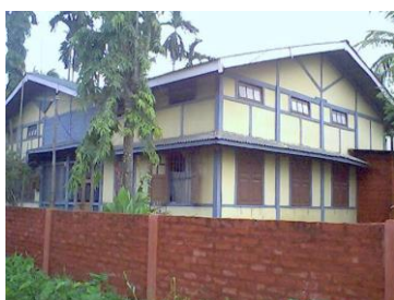
Fig. 3 Assam type houses around the city of Guwahati with typical timber framing
