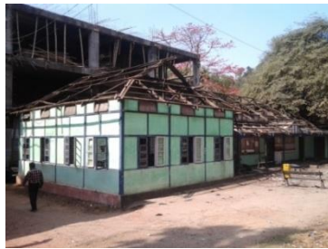
Fig. 6 Assam type house with a two-way sloped roof / hipped roof
