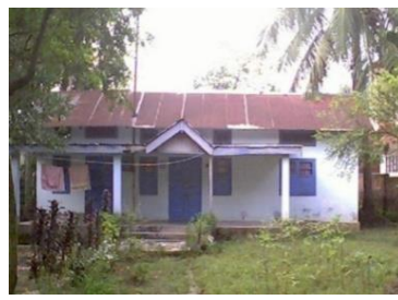
Fig. 7 Partially Unconfined masonry houses with lightweight roofing
