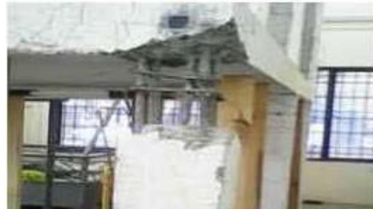
(a) The removal of spalled concrete at column bottom and at beam column joint
