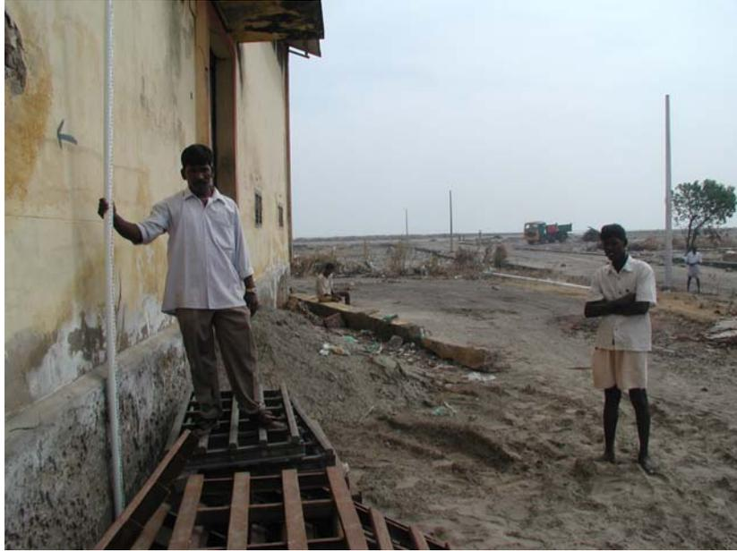
Fig. 6 Photograph of mud line at black arrow, and of flow-damaged awning at 1.2 m above the mud line, at the warehouse position 430 m in profile NAGA01 (the maximum still-water elevation, i.e. mud line, is 4.3 m MTL; the maximum surge, i.e. flow damaged awning, elevation is 5.5 m MTL; the surge elevation is confirmed by heavy debris at 5-6 m MTL in adjacent tree branches (see Figure 8); photo view direction is towards the east, with shoreline beyond view in the far background)
