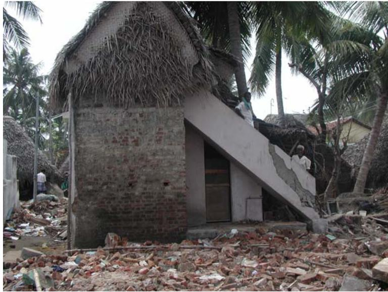
Fig. 9 Measured still-water depth (2 m) and surge depth (3 m) on a remnant standing structure in a proximal position (150 m landward of backshore) in Nagapattinam (this site is located northwest of the Nagapattinam lighthouse; rubble is from collapsed buildings adjacent to the standing structure; this neighborhood suffered substantial loss of life; photo view direction is to the south)
