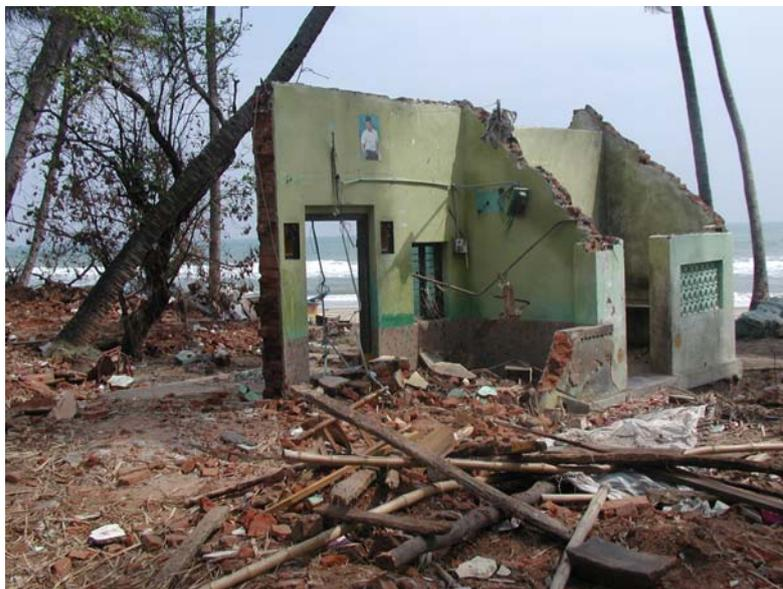
Fig. 10 Photograph of asymmetric damage and bimodal beam orientation indicating transient southwest oblique tsunami flow near profile DEVA01 (the catastrophic collapse of the trailing wall suggests that failure resulted from unbalanced internal pressures of the water-filled structure; photograph view direction is to the east; the structure is about 40 m landward from the swash zone, with shoreline visible in photo background).
