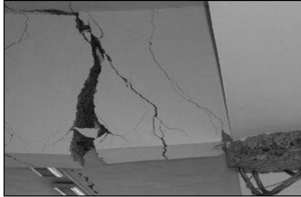
Fig. 1 Failure in a beam due to pull-out of bottom reinforcing bars (at New Passenger Terminal, Port Blair, Andaman Islands, after the earthquake in 2004)
