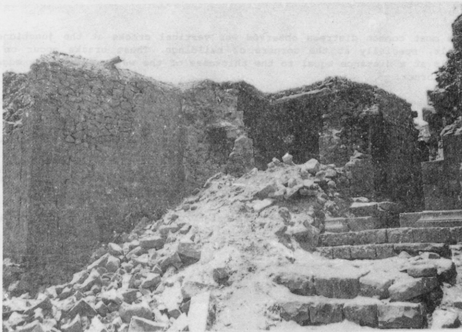
Fig.4 COMPLETE COLLAPSE OF OUTER WYTHE OF WALL
