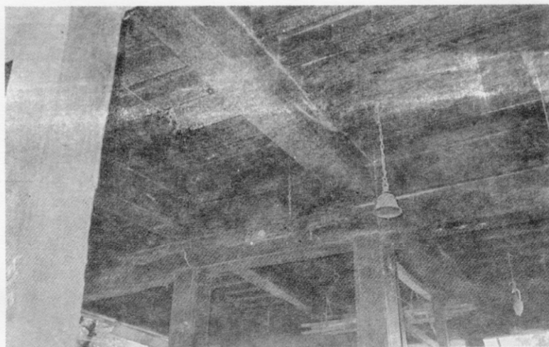
Fig 43 Inside view of roof of Ganesh temple at Sastur. The timber frame has excellent wooden joints.
