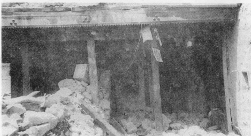
Fig 7 An old stone house with wooden frame has an intact roof at Killari. No casualties occurred in this portion of the house. Newer construction in this and adjoining houses without wood frames collapsed completely and killed the inmates.
