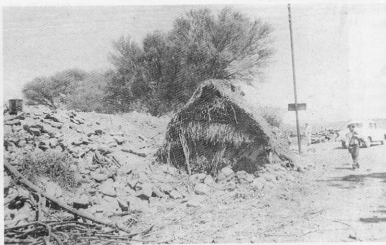
Fig 13 Huts survived but heavy stone houses collapsed.
