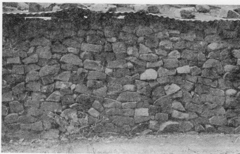
Fig 15 Dry pack masonry with big sized stones, in rural houses of Karnataka.
