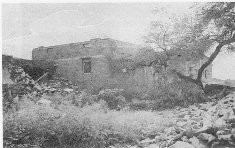
Fig 18 An undamaged building with RCC bands at Killari, surrounded by collapsed stone houses.
