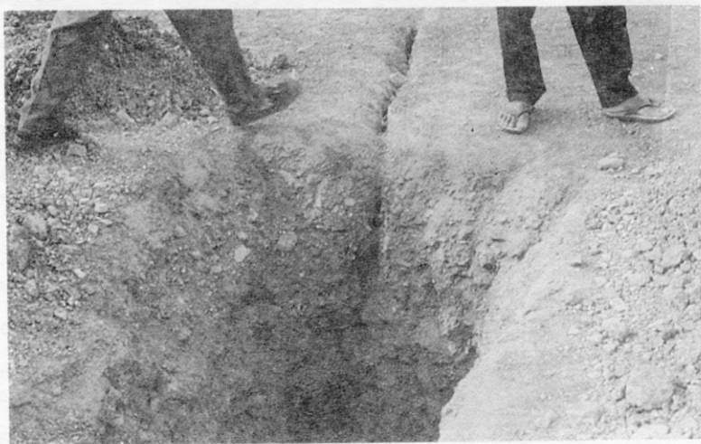
Fig 23 One meter deep fissure in left embankment of lower Terna dam, as confirmed by pit opening.
