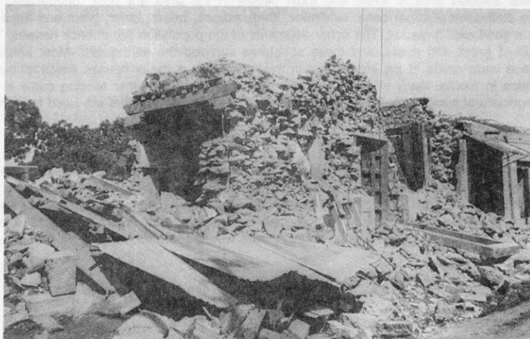
Fig 3 This heap of stone rubble, timber and mud was street of stone houses at Killari before the earthquake.
