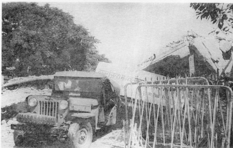
Fig 9 A jeep trapped under the collapsed RCC roof of District Cooperative Bank at Killari. The RCC roof rested on stone walls before the earthquake.
