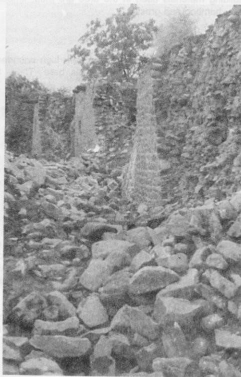
Fig 4 Failure of stone wall. The outer wythe bulged out and collapsed completely, Sastur.
