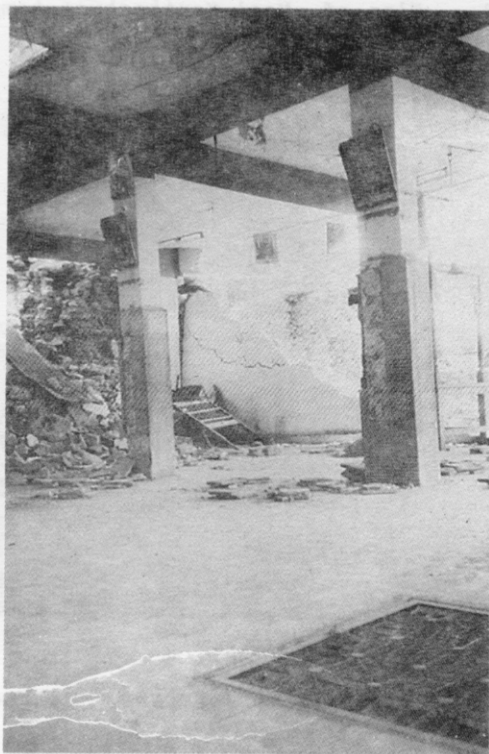
Fig 41 Undamaged RCC frame at Neelkantheshwar temple, Killari. Tiles fixed on RCC column fell off.
