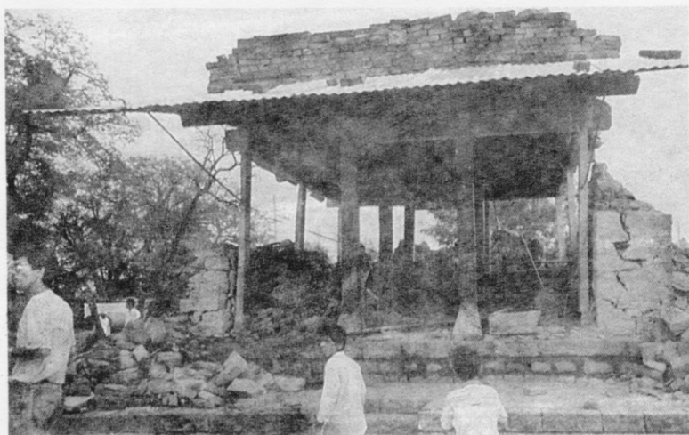
Fig 42 Ganesh temple at Sastur. Walls around the timber frame collapsed outwards while the roof is intact.
