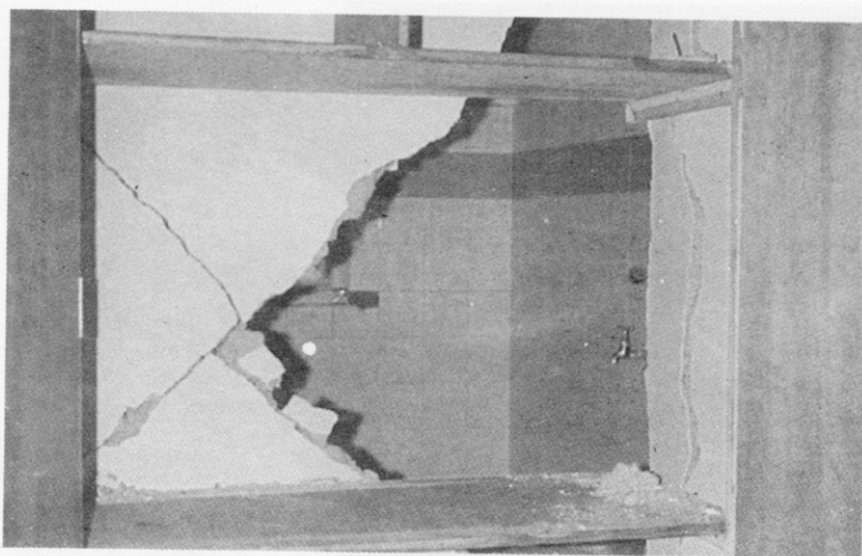
Fig 25 In the brick masonry building of rest house of Lower Terna Dam Project at Makni, walls cracked, plaster fell off from walls and part of a half brick thick partition wall collapsed. Fig shows a portion of the collapsed partition wall between bedroom and washroom.
