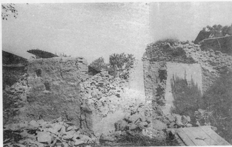
Fig 12 Collapsed adobe house at Killari.
