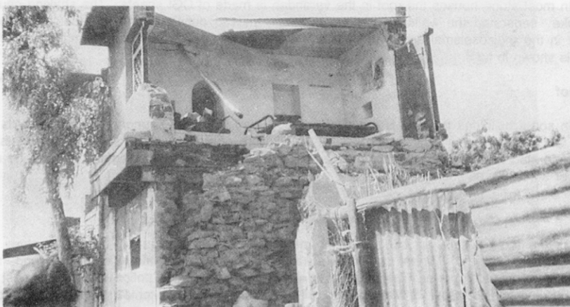
Fig 6 Failure in a construction of mixed type at Killari. Brick was laid in cement-sand mortar to make walls above a stone house. The brick wall slid and came down en masse as there was no connection between old and new type of construction.
