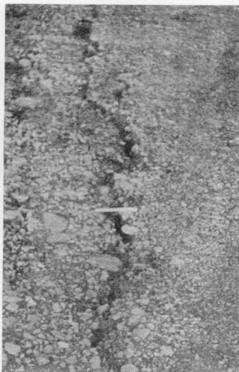
Fig 21 Fissure in left embankment of canal near Ganjankheda.
