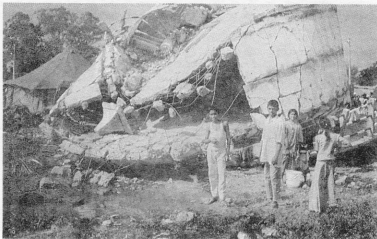
Fig 26 Failed overhead water tank with domical base at Kawtha.
