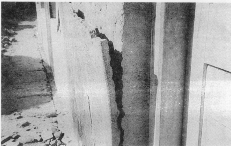
Fig 31 Thick plaster bulged out at Dr. Bhujbal's clinic, Killari.
