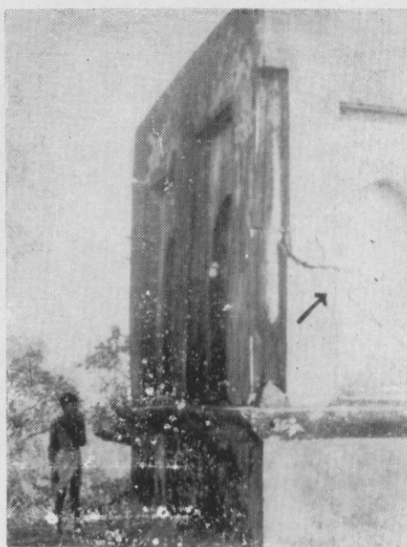
Fig. 27. Damage to a very old Shiva temple in brick masonry.
