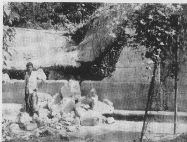
Fig. 4. Mud house at Chotamamda with thatched roof whose collapse of a wall led to death of three persons inside-this is one of those few examples where the roof had also been broken.
