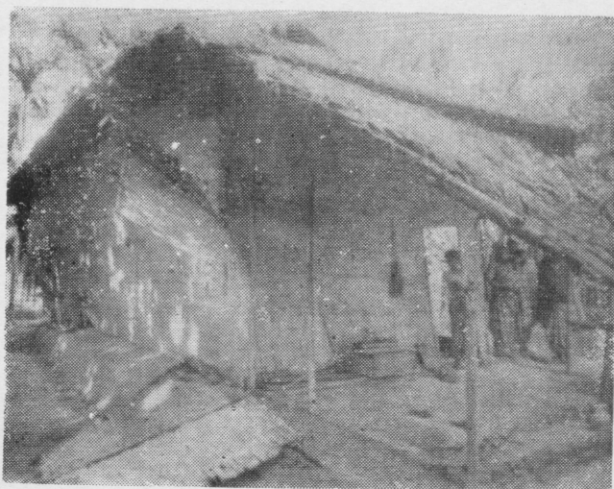
Fig. 8. A thached hut with walls in bamboo mat and mud plaster is tilted and mud plaster is partly peeled off.
