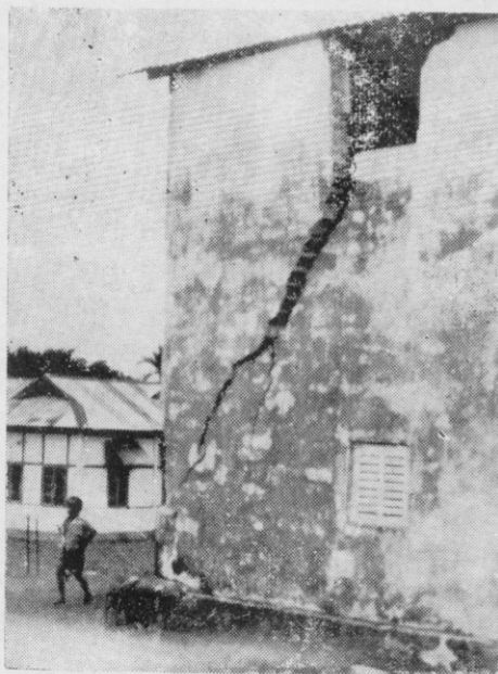
Fig. 21. Damage to a tubular steel frame shed with brick masonry filler walls-the steel-barties have served as hinges for the broken wall.
