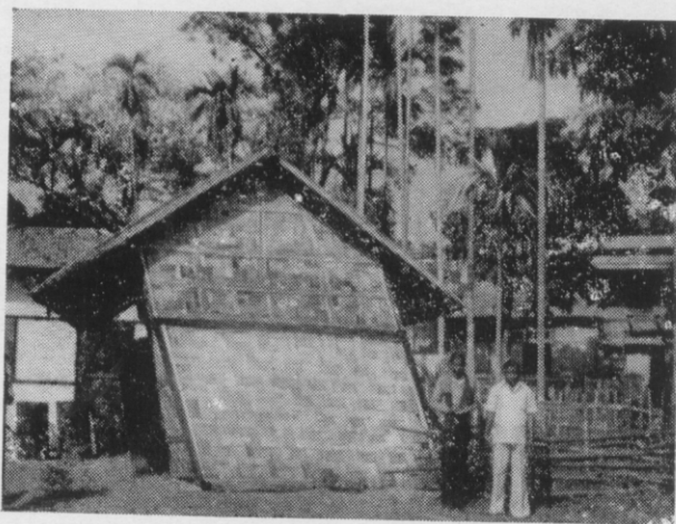
Fig. 10. Tilting of a very light hut in timber and bamboo at the compound of Sonaimukh inspection house.
