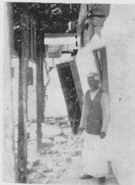
Fig. 13. Very extensive damage to a timber cum brick masonry building of school at Sonaimukh-the tilted door hangs with masonry due to lintel level reinforcement.
