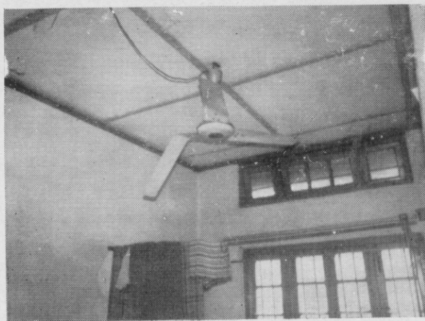
Fig. 24. Banding of fan blades in the building in figure 23-some evidences of slipping of false ceiling attached to roof above the ventilator were seen.
