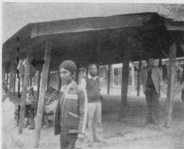
Fig. 6. 30 × 10m timber shed for daily market at Sonaimukh was tilted by about 30° market is being restored to verticality.
