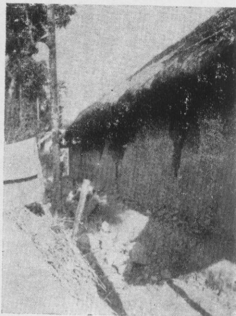
Fig. 3 A mud house at Sonaimukh whose longer wall has been damaged-cracks have travelled from the openings more or less vertically perhaps top to bottom.
