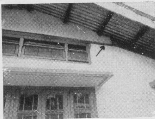
Fig. 25. Close up of the slide surface between ceiling and walls of the building in figures 23 and 24.
