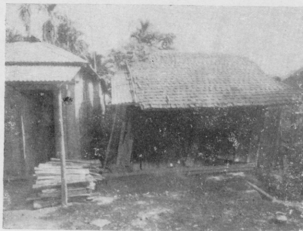
Fig. 11. Tilting of yet another individual shop with roof in tiles.
