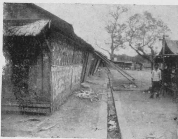
Fig. 9. Tilting of a row of shops in the Sonaimukh market-efforts to restore them to vertical by giving supports as in photograph were already in progress.
