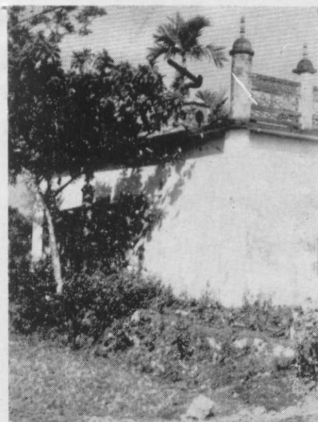
Fig. 28. Collapse of the rear parapet over the roof in a mosque at Kajidhar II.
