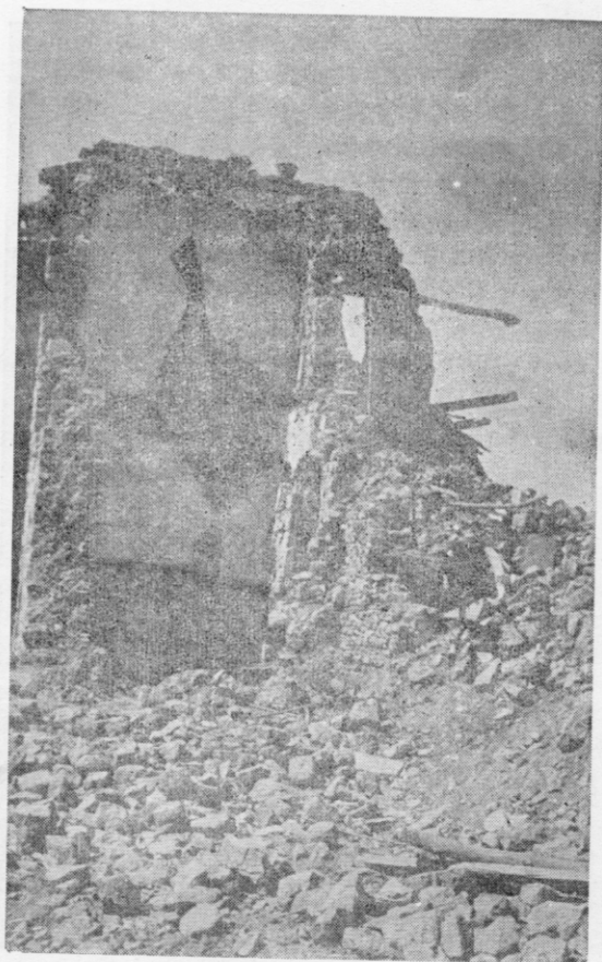
Photo 6. Complete Collapse of a house of random stone construction with muck filling in the hearting of walls at village Dohran.
