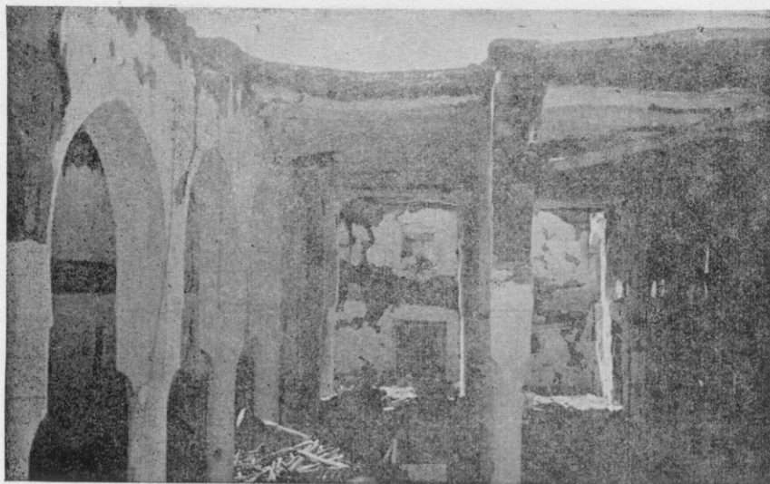
Photo 11. Damages to the Dohran Madarsa-cum-Mosque, fallen wood pieces from roof, cracked and peeled off plaster on walls and pillars.
