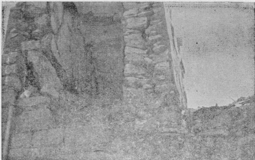
Photo 13. Random rubble stone wall, no interlocking between inner outer faces of stones at Village Hizrat Mangada.
