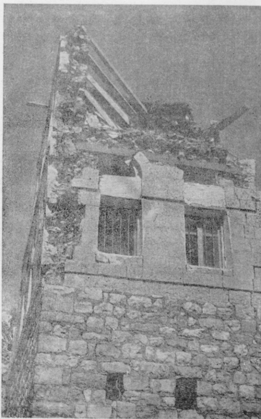
Photo 8. Collapse of third storey and cracks in lower storey walls, very heavy floors in houses seen in village Dohran.
