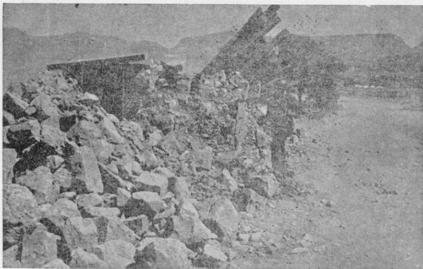
Photo 3. Complete Collapse of a single storied dwelling of random stone construction near Dohran.
