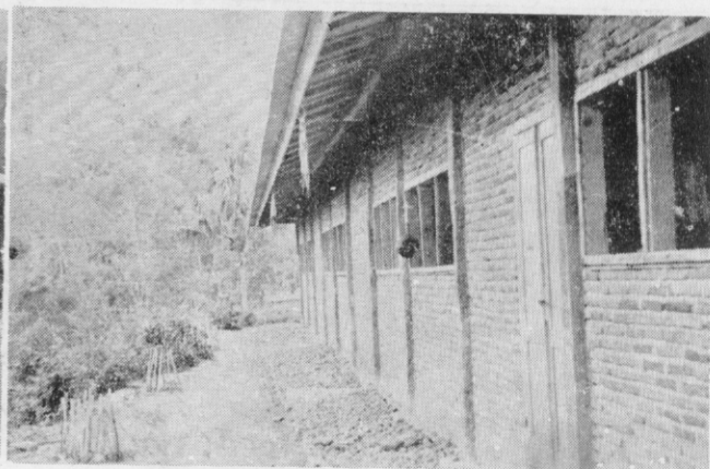
Photo 11, 12 Primary school at Gitgit, Bali. Indonesia New construction after July 1976 earthquake. RC posts under each wooden truss, Ring beam at plinth, none at lintel or eave level, Brick wall panels, brick, gable, Quality of construction substandard
