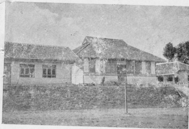
Photo 9. School Buliding off Bandung. Indonesia old building at centre has ring at plinth level, Buliding at left, new addition, has no such provision.
