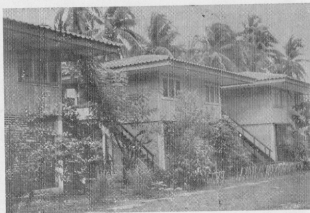
Photo 19. Two storey Teachers' Houses, Bangkok, Thailand. Lower storey, RC posts, brick walls. Upper storey, timber floor joists & planks, timber posts & roofing system.
