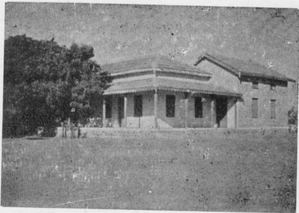
Photo 7. Primary School at Anjar, Random rubble masonry construction, has no strengthening provisions for seismic forces, no damage to the building in 1956 Anjar Earthquake to good construction.
