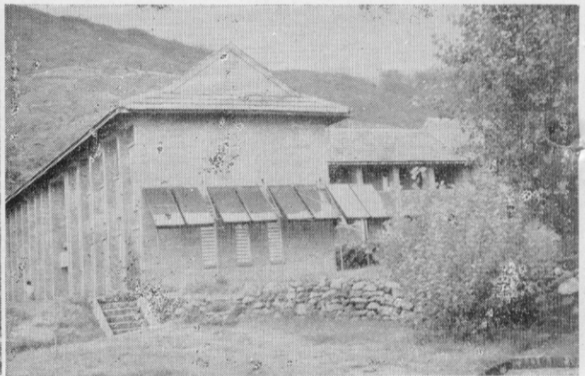
Photo 15. British Aided School in Kathmandu, Nepal. Good quality brick construction with RC ring beams, slab and beam floors (inclined plates are for collecting solar heat for water heating).
