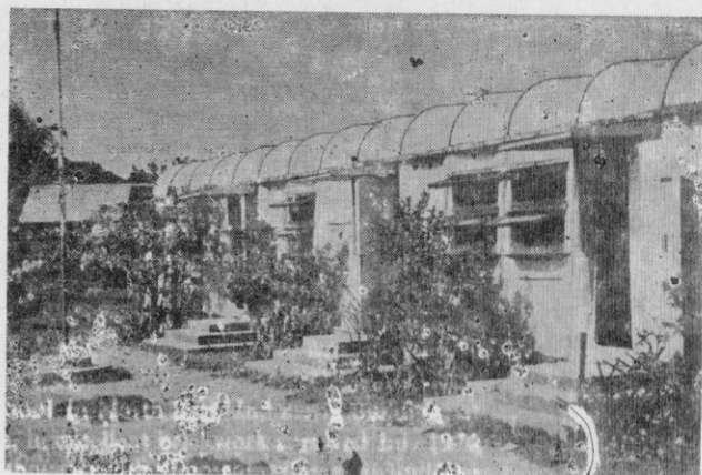
Photo 2 Government Primary School, East Khilgaon, Dacca, Bangladesh. Long sides and roof of jute plastic, ends brick wall upto eave level (too hot, but no corrosion problem in coastal areas).
