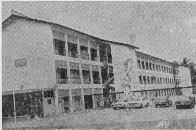
Photo 13. National Secondary School, Kuala Lumpur. Malaysia RC Frame Building with Wooden truss roof. Stair block separate, structurally connected at roof level.
