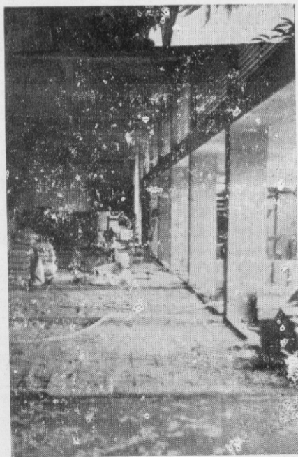
Photo 18. Four storey school construction, Bangkok, Thailand. RC frame building, pile foundations. RC beams at plinth level bothways seen in the photo.
