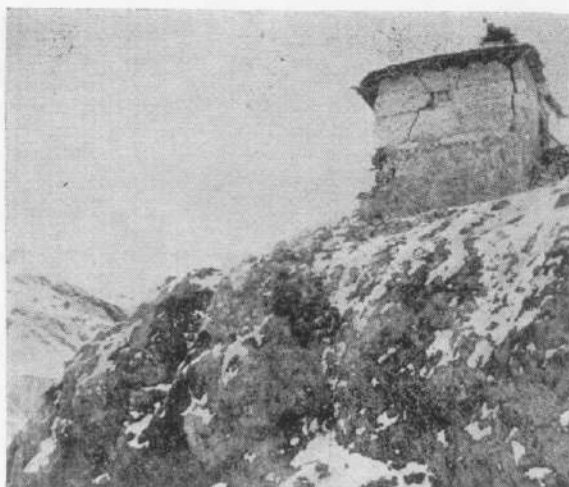
Fig. 18. Severe damage to the priest's house at Shalkar village.
