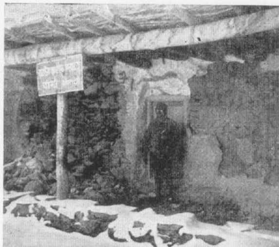
Fig. 24. Failure of RRSM interior walls of the primary school building at Chango village.
