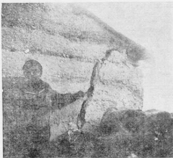
Fig. 4. Cracks in mud house at Pinauti village.
