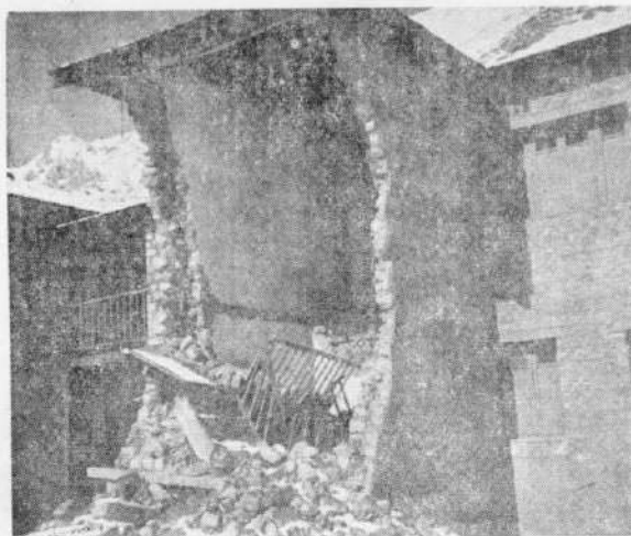
Fig. 33. Collapse of staircase well on the rear of the police station building at Leo village.
