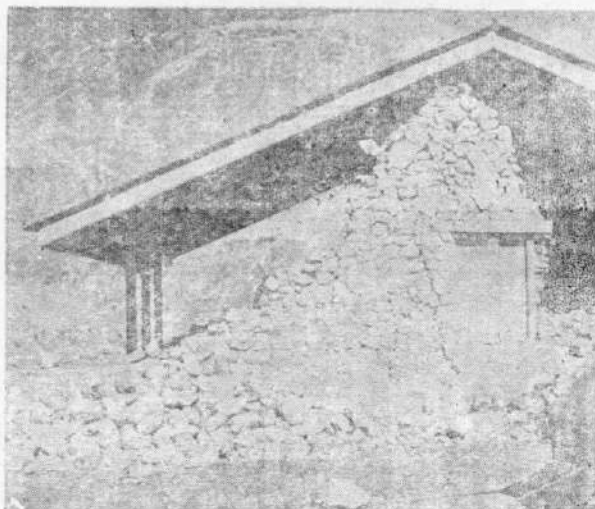
Fig 9. Damage to gable end wall of P. W. D. rest house at Sumdoh village.
