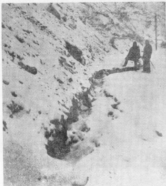
Fig. 76. Fissures parallel to the road on glacial moraine hill side between Malling and Chango.
