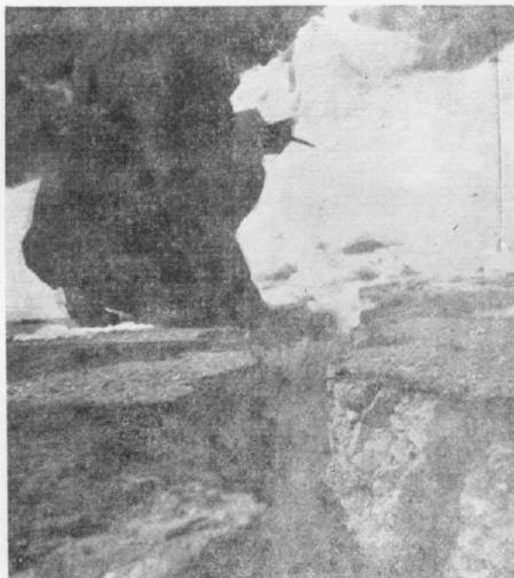
Fig. 54. Ground fissures transverse to the road with openings upto 60 cm in width between Sumdoh and Kaurik. The extension of the fissure in the hill mass covered with snow is seen in the background.
