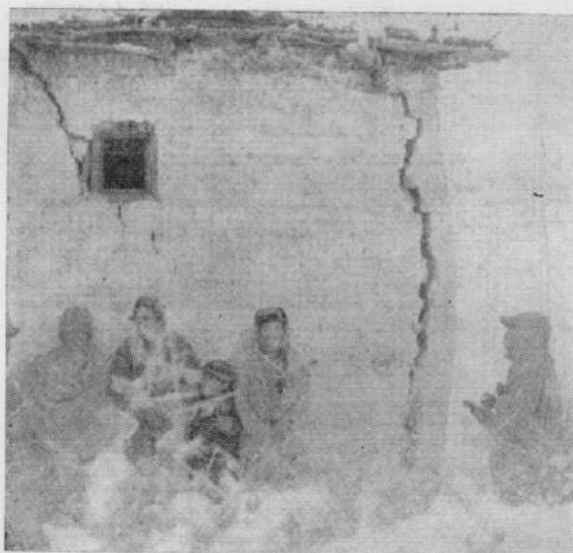
Fig. 23. Bulging of the end wall and cracks propagating from window openings of a mud brick house at Chango village.
