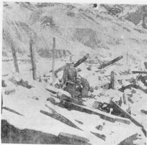
Fig. 20. Total collapse of timber frame work of a temple at Shalkar village. The Buddha idol is also damaged.
