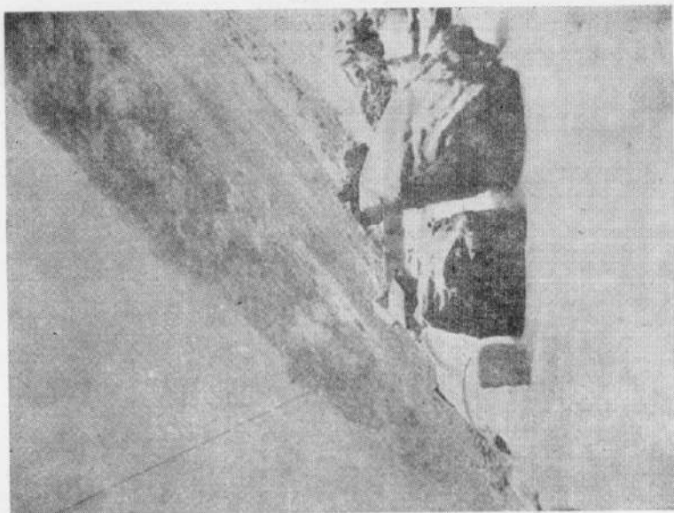
Fig. 73. Huge boulders fallen on road pavement between Malling and Chango. A huge landslide is seen in the back-ground which has washed out the road completely.
