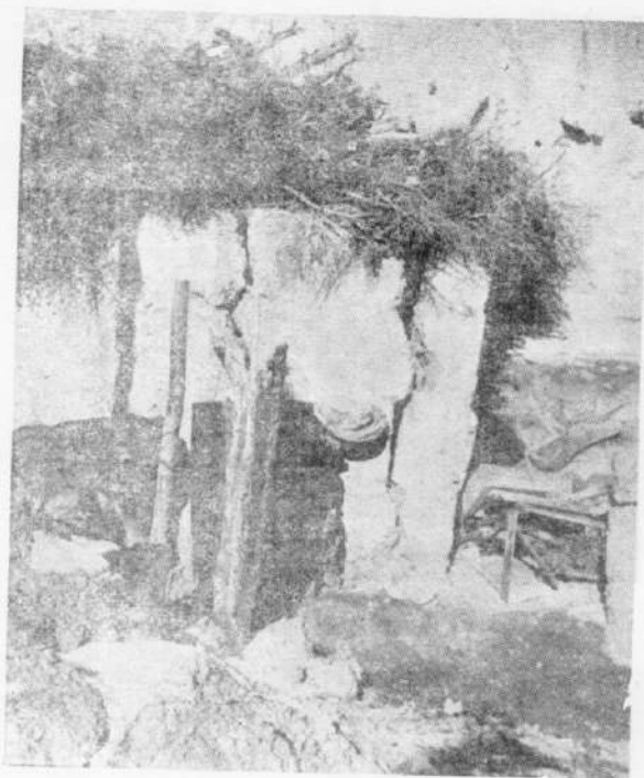
Fig. 6. Collapse and fall of a house made of cast insitu mud walls at Kaurik village.
