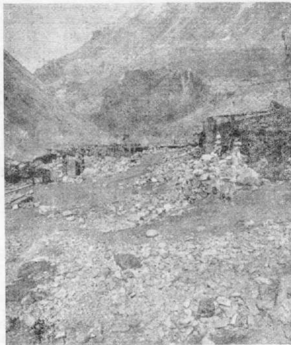
Fig. 8. Collapsed RRSM houses at Sumdoh village.
