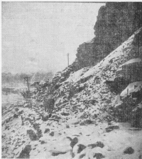
Fig. 66. Rock slides in quartzites along H.T. road between Chango and Shalkar.
