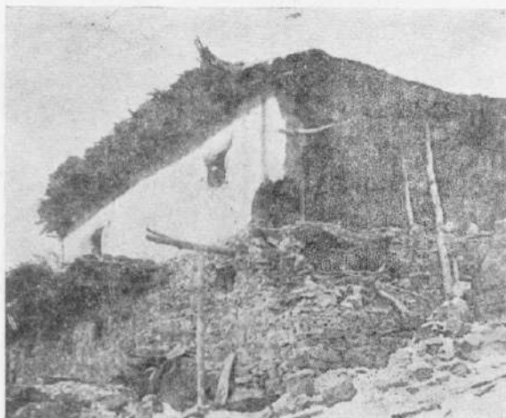
Fig. 16. Complete collapse of E-W wall of mud brick of a double storey house at Shalkar village. The ground floor is in RRS in mud mortar.
