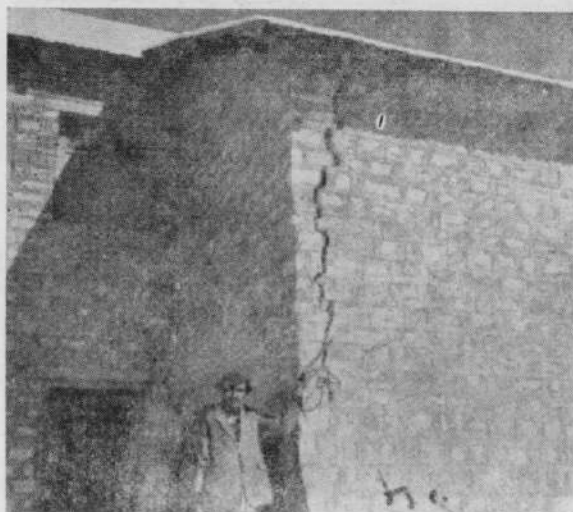
Fig. 36. Vertical cracks at the junction of walls in Ayurvedic hospital at Leo village,
