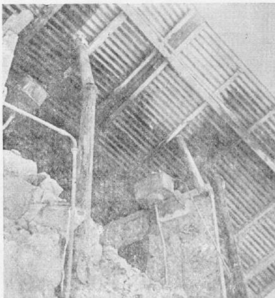
Fig. 32. Collapse of gable end wall in a house at Leo village. A timber frame interior wall with stone masonry filler built in Kashmir Dhaji-Dewari type construction did not collapse. Movement of the roof resulted in tilting and dislocation of sewage ventilation pipes.
