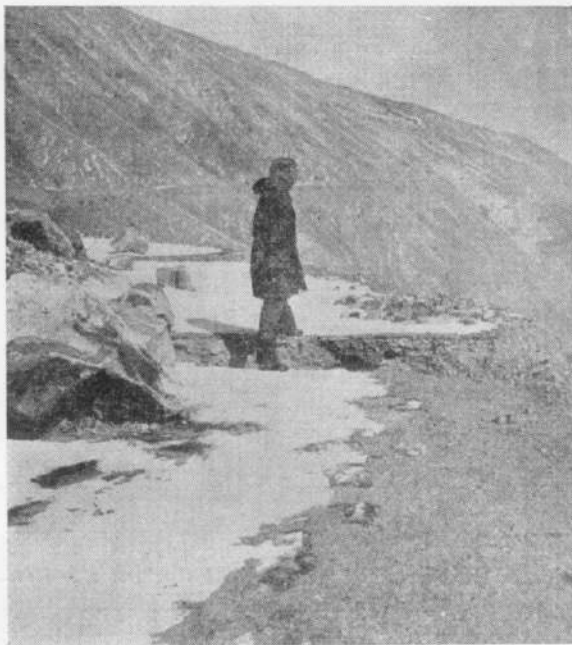
Fig. 53. Step faulting with down throw side towards west on Hindustan Tibet road between Sumdoh and Kaurik.
