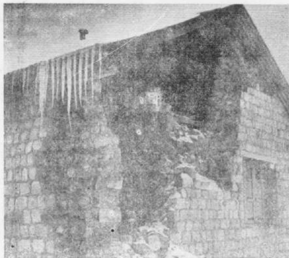
Fig. 26. Collapse of stone masonry gable end wall in Patwarikhana, at Chango village. Dressed stone was used in the outer facings whereas random rubble stone was used in the inner facings with muck filled in between,
