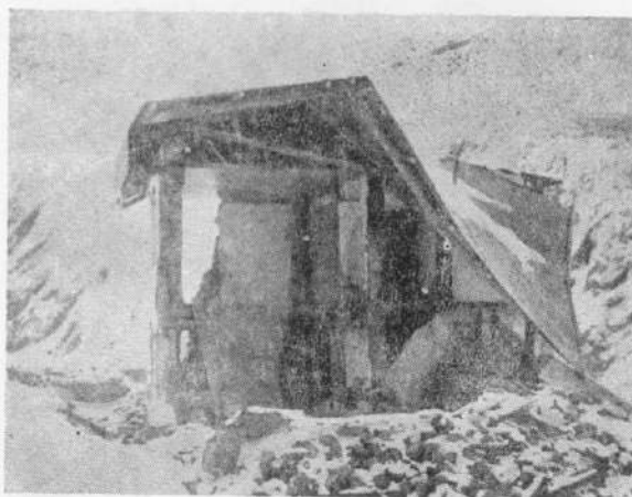
Fig. 17. Collapse of police check post at Hindustan Tibet road, Shalkar. A big boulder rolling down from left seen below the collapsed roof, caused severe damage to the building.
