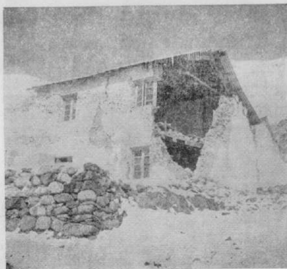
Fig. 37. Collapse of gable end wall of two storeyed compounder's residence at Leo village. Fall of mud plaster can be seen on the walls.
