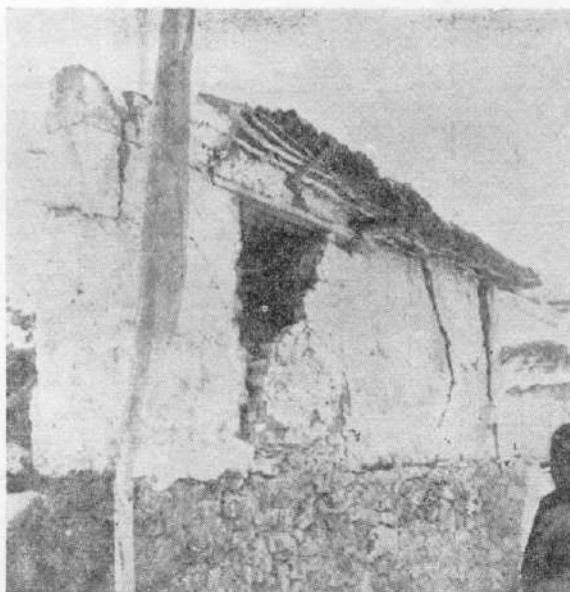
Fig. 15. A badly damaged wall resting on plinth of RRSM without mortar. (All other walls of the house have collapsed) at Shalkar village.
