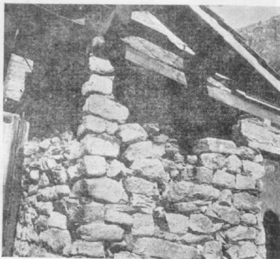
Fig. 45. A house with RRSW without mortar suffered heavy damage at Tapri village.
