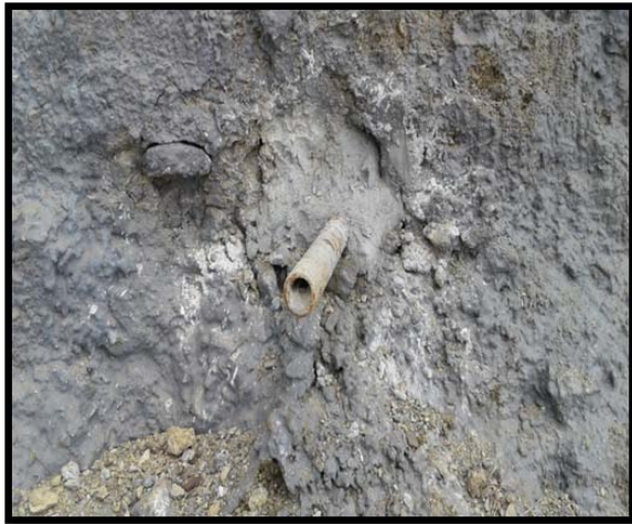
Fig. 8 (a): A view of self drilling anchor
