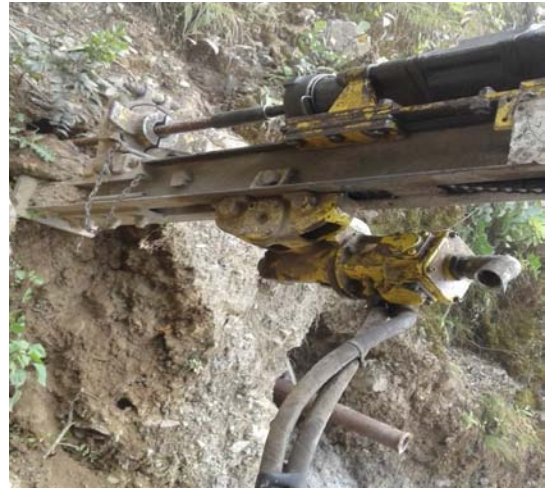
Fig. 8 (b): Special machine for driving Self drilling anchor
