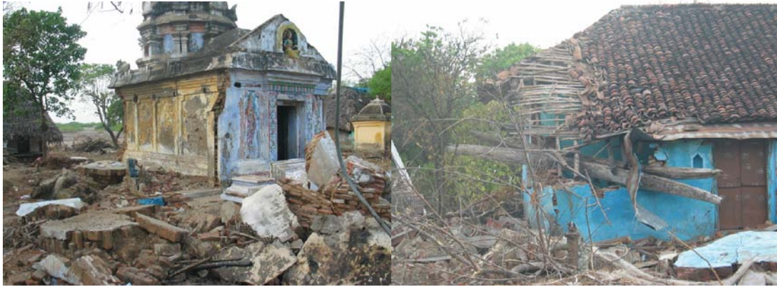
Fig. 13 Damage to small houses in Kuddupattanam (south of Chidambaram), Nagappattinam
