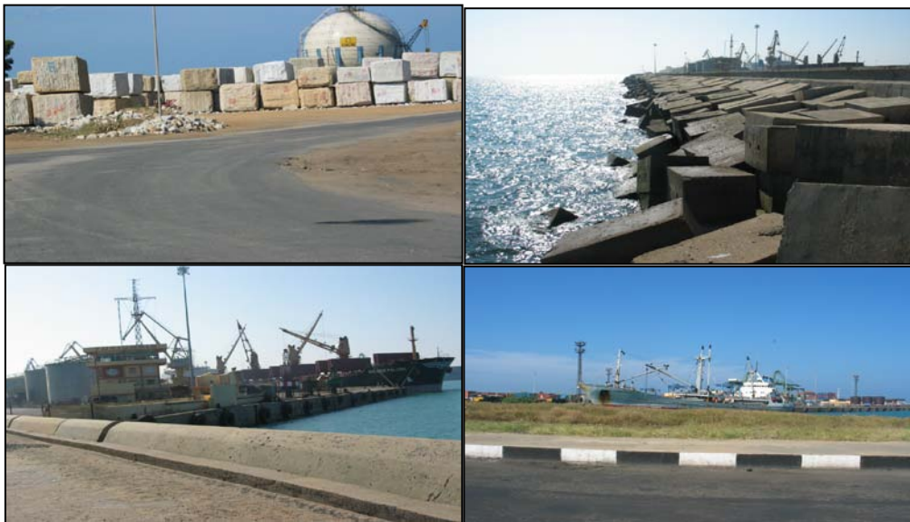
Fig. 22 Pictures taken at Tuticorin harbor showing no damage to the facilities there and life remaining normal at the port (clockwise from top left: an oil storage tank; very heavy stones (about 10 tonnes each) to protect the break-water; a ship moored near the seashore; close-up view of another ship)
