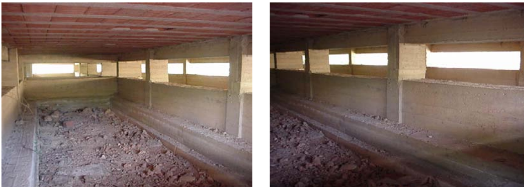
Fig. 16 Foundations of an IACP building in Solarino
