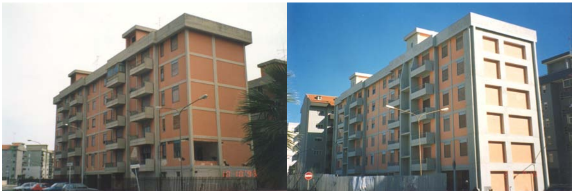
Fig. 10 Building owned by IACP of Syracuse in the Saline district of Augusta (seismic retrofitting by increment of strength and stiffness provided by newly inserted reinforced concrete cores)
