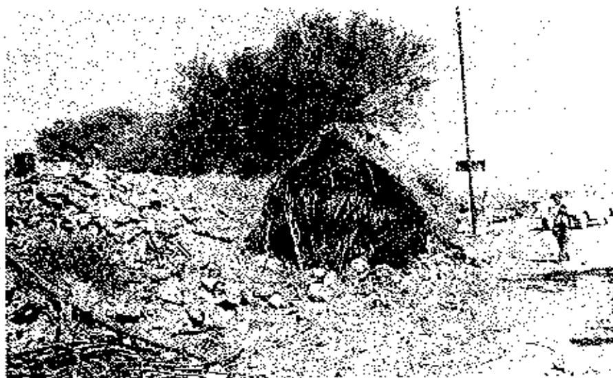
Fig 13 Huts survived but heavy stone houses collapsed.
