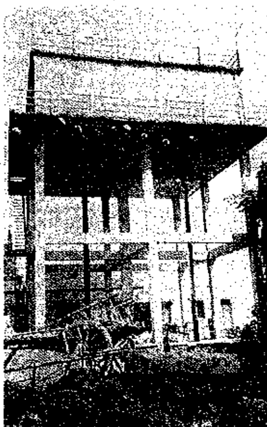
Fig 29 Undamaged water tank at Killari.
