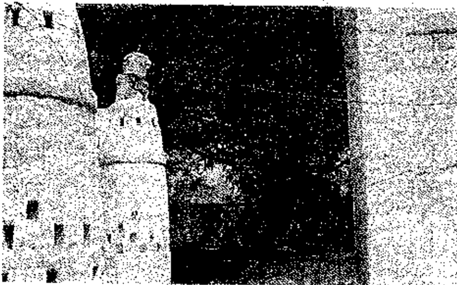
Fig 47 Damaged minaret of mosque at Kharosa.
