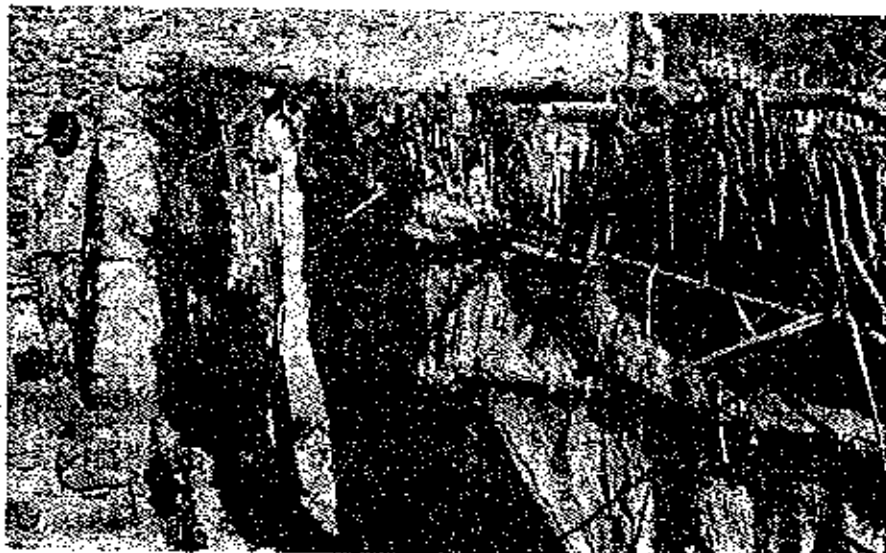
Fig 14 Reed coated with mud, Killari.
