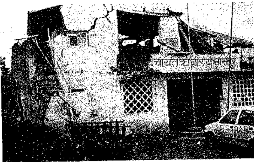
Fig 10 Brick building of Panchayat office at Sastur showed extensive damage to the first floor. This was because the tin roof rested on iron rafters and did not have a roof band.
