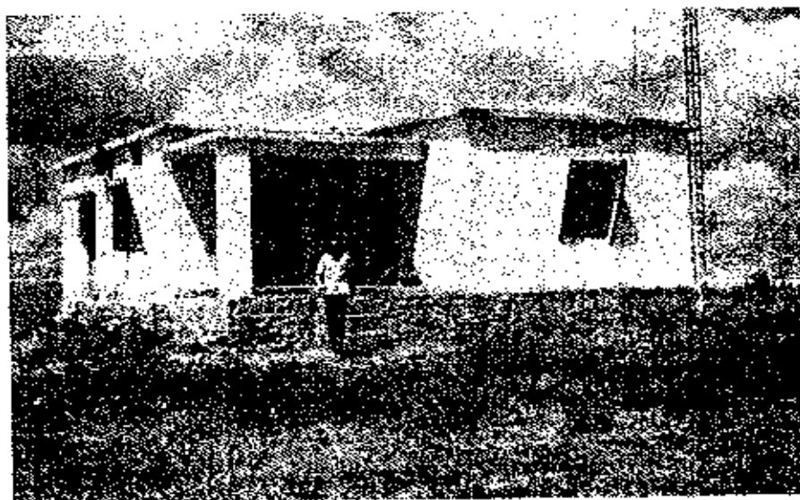
Fig 48 Intact wireless building on hillock at Kharosa.
