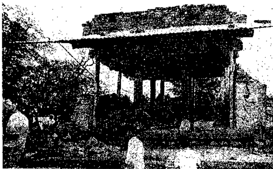
Fig 42 Ganesh temple at Sastur. Walls around the timber frame collapsed outwards while the roof is intact.
