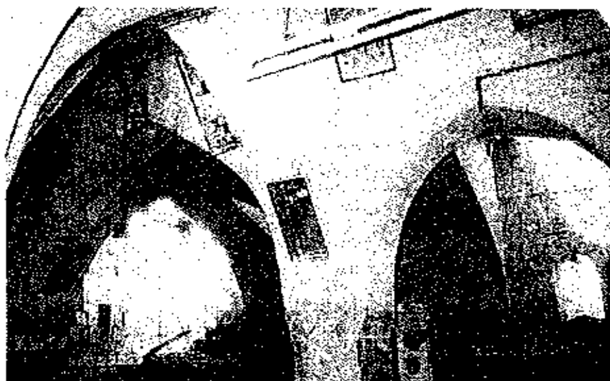
Fig 40 Worship place with arches and RCC roof at Neel Kantheshwar temple, Killari. This portion of the temple survived with minor cracks in arches.
