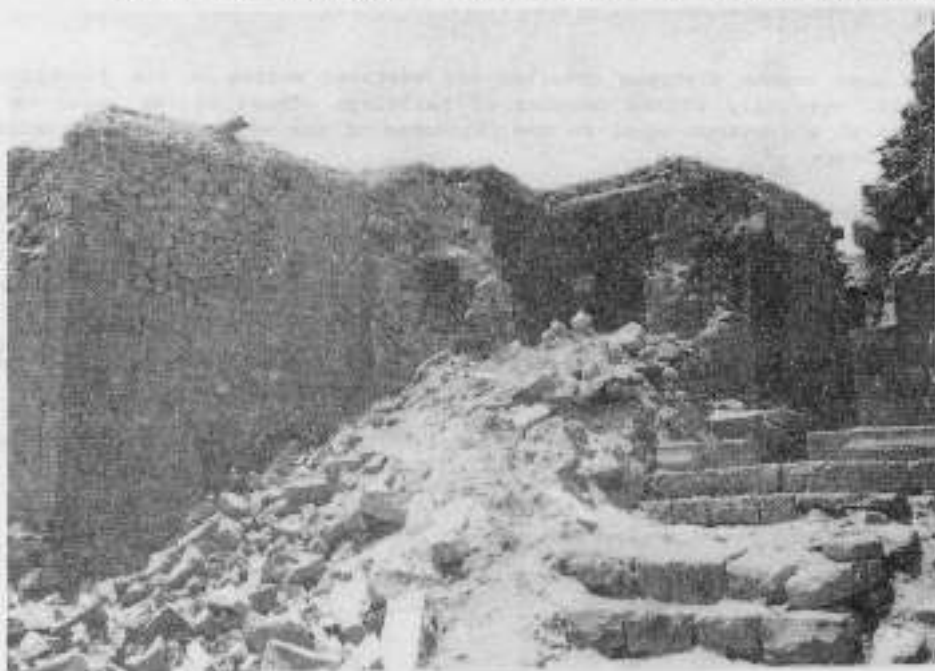
Fig.4 COMPLETE COLLAPSE OF OUTER MASONRY OF WALL
