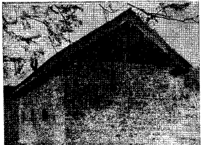
Fig. 38. Undamaged Coursed Rubble Masonry Construction with a Timber Runner at Lintel level in Mir Maidan.
