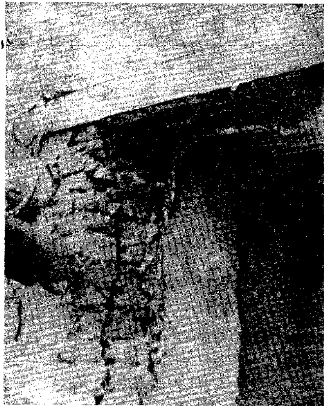
Fig. 9. Longitudinal Section of an Adobe Pier
