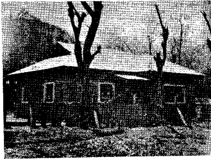
Fig. 39. Undamaged Random Rubble Masonry House in Verinag with a Lintel Band
