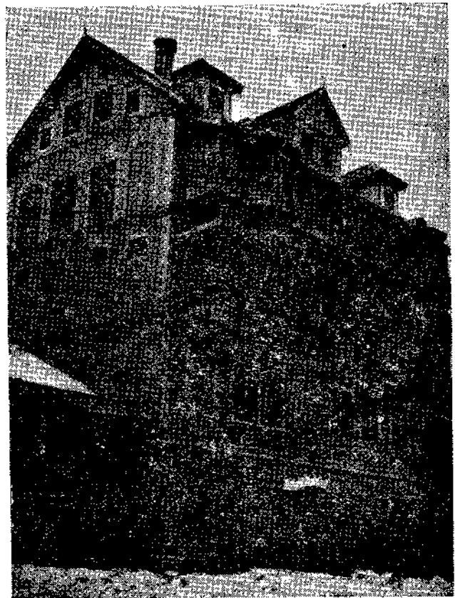
Fig. 42. Undamaged Four Storey Building in Anantnag.
