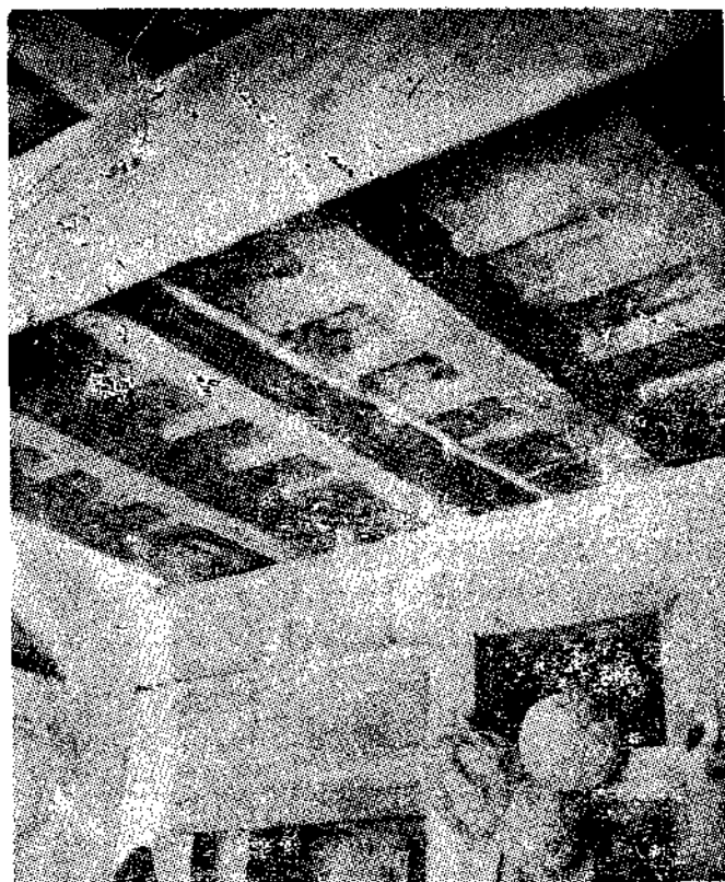
Fig. 13. Common Roofing System in a "Dhajji-Diwari"
