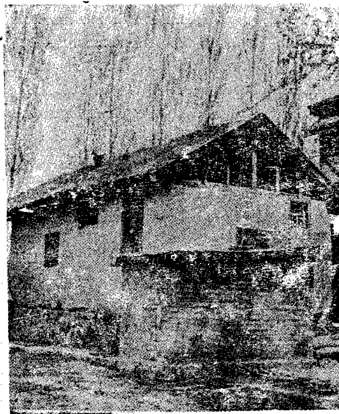
Fig. 14. "Dhajji-Diwari" with a Birch Bark Roof
