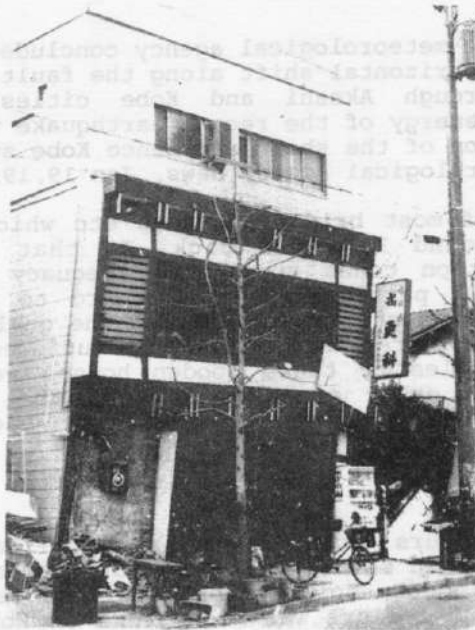
Fig.3 Typical wood house failure
