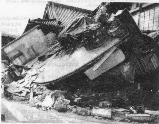
Fig.4 House failure due to heavy roof
