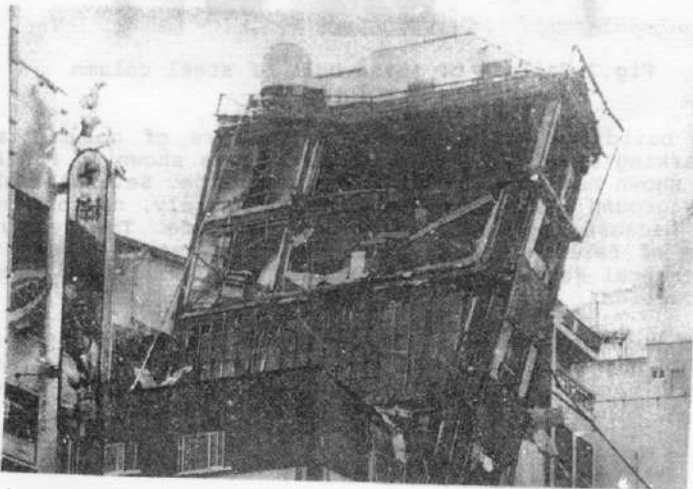
Fig.6 Failure of steel frame structure due to large ductile deformation
