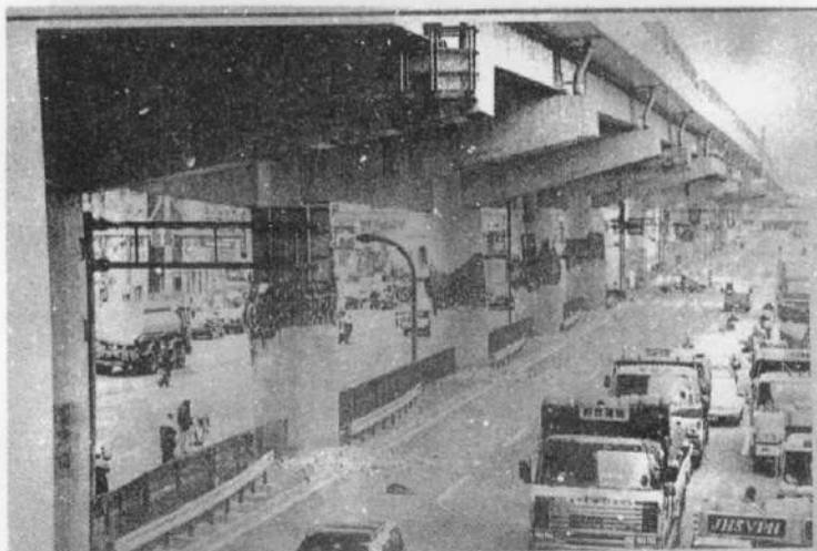
Fig.14 Failure of columns of highway due to compression
