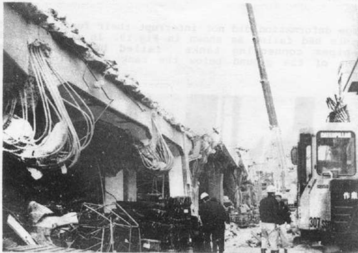
Fig.17 Failure of columns of train parking stand due to compression (Kobe city)
