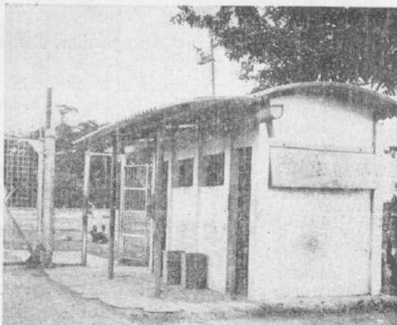
Fig. 18. The Watch and Ward Post, at Henry's Shaft Gate in prefabricated reinforced concrete construction, which did not suffer any damage.
