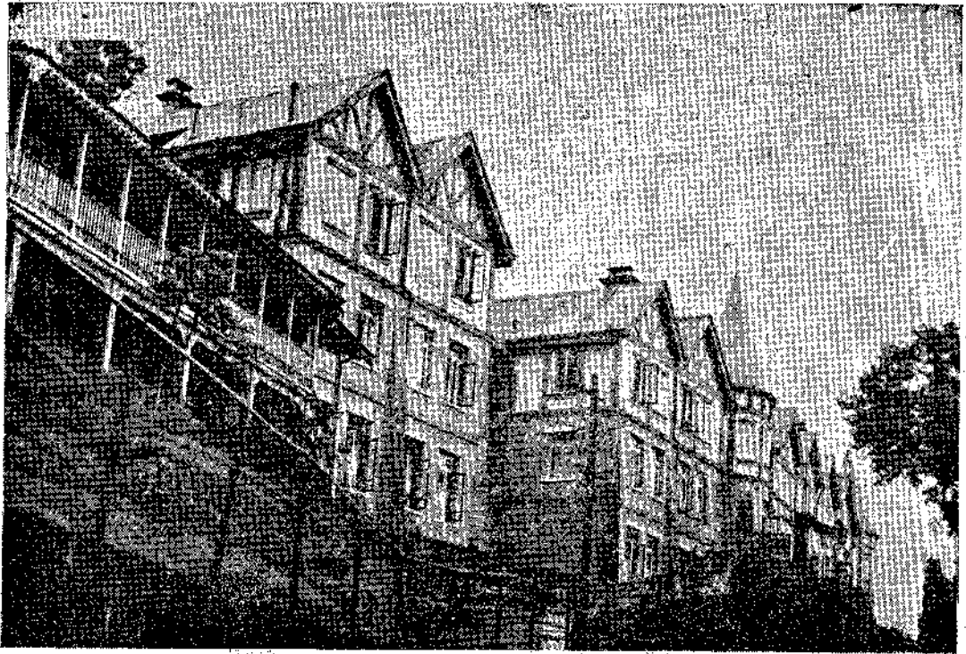
Fig. 9 Stone Masonry Buttressed Walls of Mt. Everest Hotel, Darjeeling
