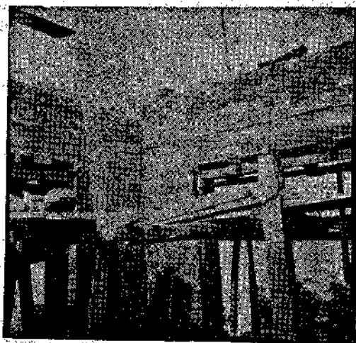
Fig. 11 Continuous Lintel Band in Stone Masonry Wall.
