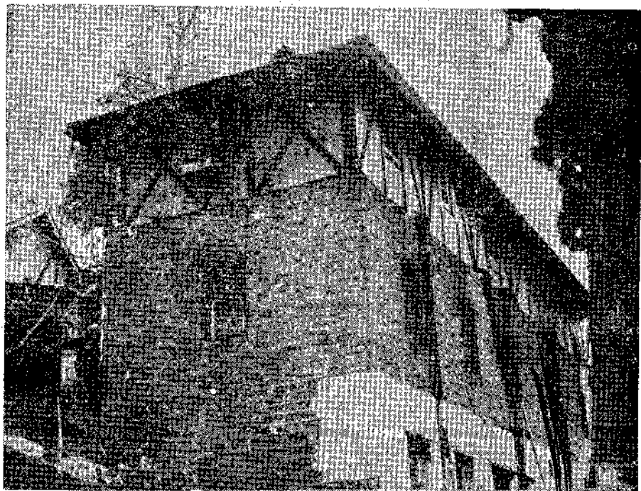
Fig. 10 Stone Masonry and Metal Lath-Plaster Construction, Darjeeling.
