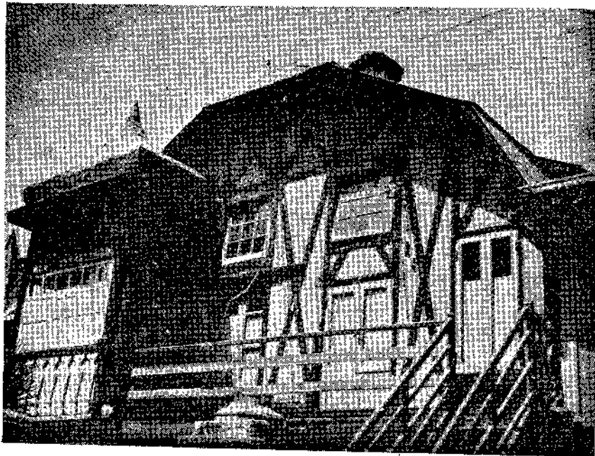
Fig. 8 Brick-nogged Building in Darjeeling.
