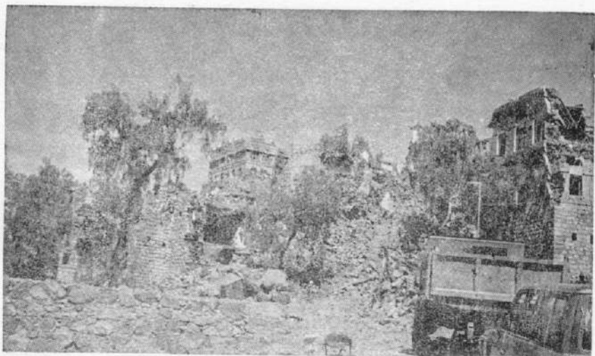
Photo 22. Destruction of houses in village Dohran.
