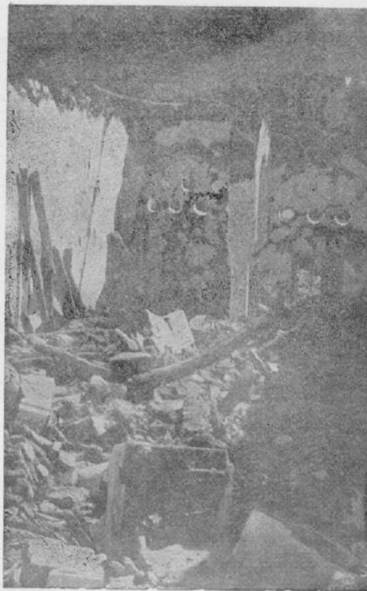
Photo 9. Collapse of Dohran Mādarsa-cum-Mosque, some Arches and posts still standing.
