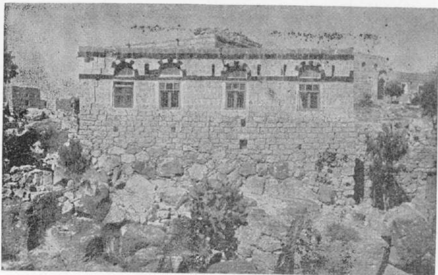
Photo 17. Random stone and coursed stone construction, cracks and separation at corner of wall at Village Hizrat Mangada.
