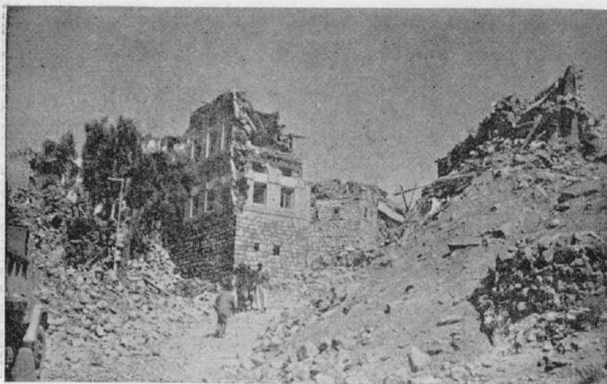
Photo 7. Collapse of stone built dwellings in village Dohran.
