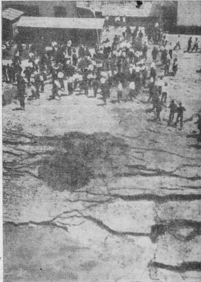
Fig. 1. Initial Stages of the Water Flow from Ground, Niigata (1964)
