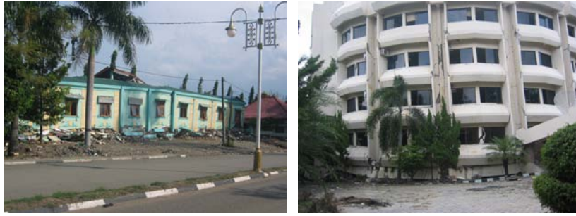
Fig. 28 Soft story failures in Banda Aceh
