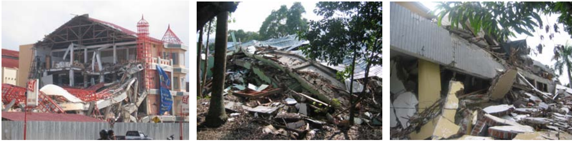
Fig. 11 Earthquake damage in Banda Aceh, Indonesia
