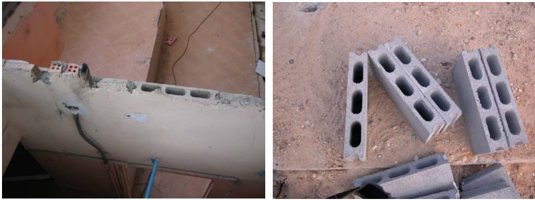
Fig. 15 Clay brick and concrete masonry block units with 50 mm thickness
