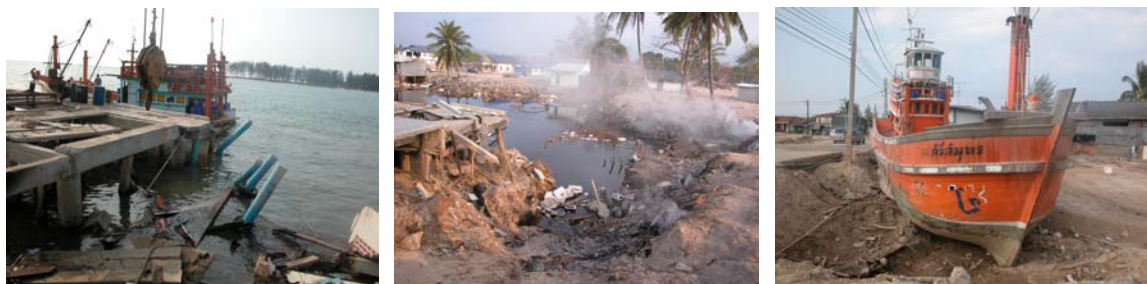
Fig. 8 Damage to Khao Lak harbor town
