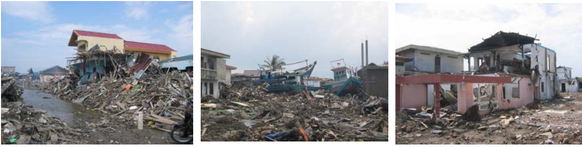
Fig. 10 Tsunami damage in Banda Aceh, Indonesia
