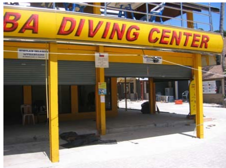
Fig. 22 Steel frame structure in Phi Phi Island
