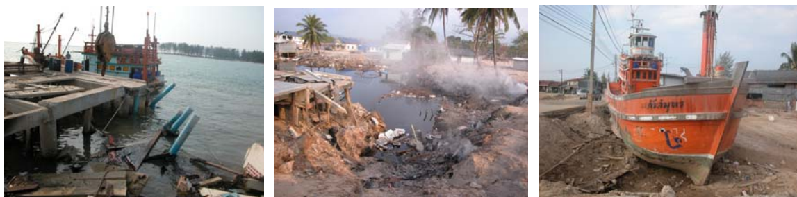
Fig. 8 Damage to Khao Lak harbor town
