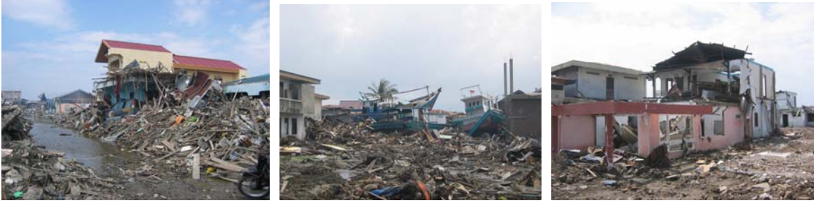
Fig. 10 Tsunami damage in Banda Aceh, Indonesia
