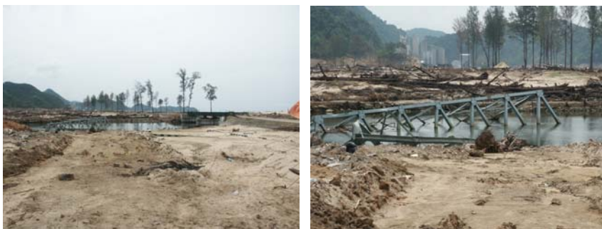
Fig. 23 The failure of steel truss bridge in eastern Banda Aceh
