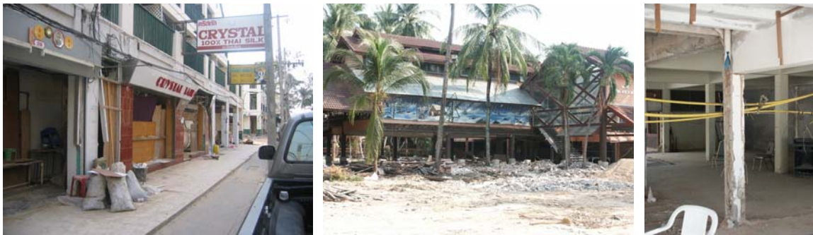
Fig. 5 Damage in Patong Beach
