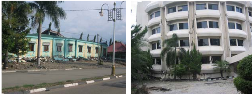
Fig. 28 Soft story failures in Banda Aceh
