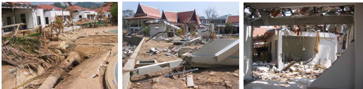
Fig. 7 Structural and nonstructural damage in Khao Lak Beach
