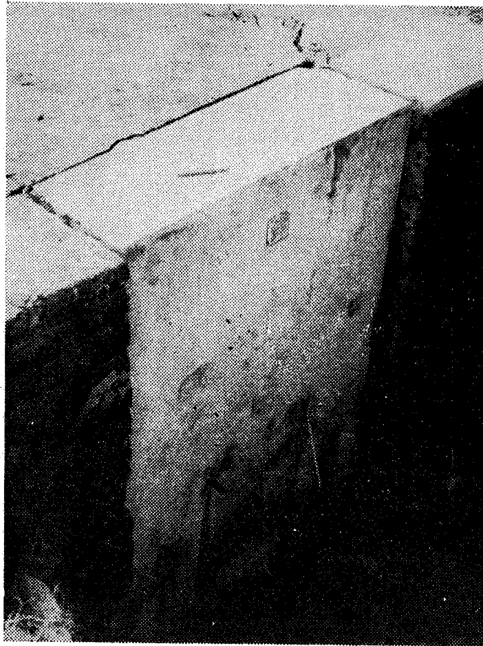
Fig. 7. Crack pattern after passive pressure test.
